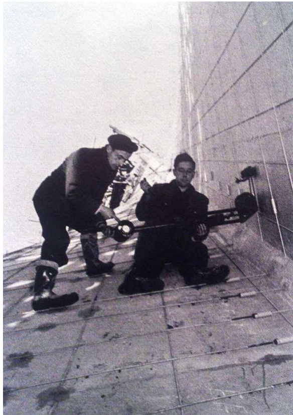
Figure 28 auxiliary devices used to apply the pre-stressing
